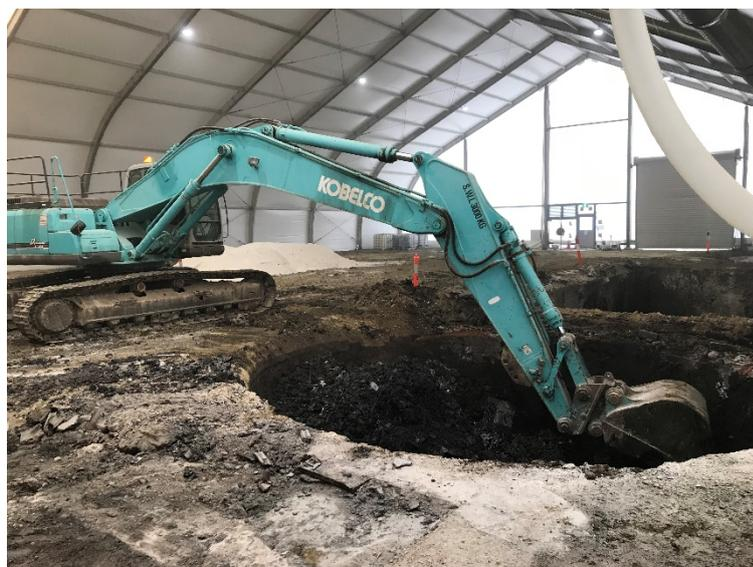
Figure 2: Excavation of Tar Pit within Odour Control Enclosure
